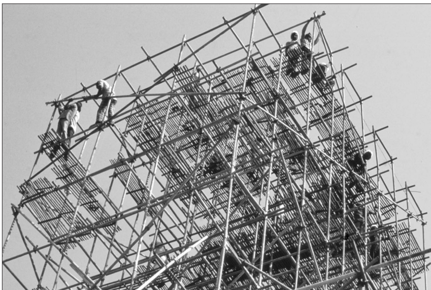
Construction of scaffolding in New Delhi (Photographer: J Maillard. Copyright: ILD)
